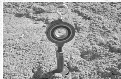
Insert pivot bearing in the tube. Use the two nuts to adjust the height for the center of the pour. The top of the pour is 3/8 inch up from the bottom edge of the pivot bearing nut. Tighten the two nuts against each other at the correct height.
