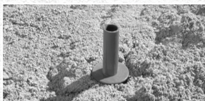
Drive centering tube into the centerpoint of the pour up to the stop flange.
